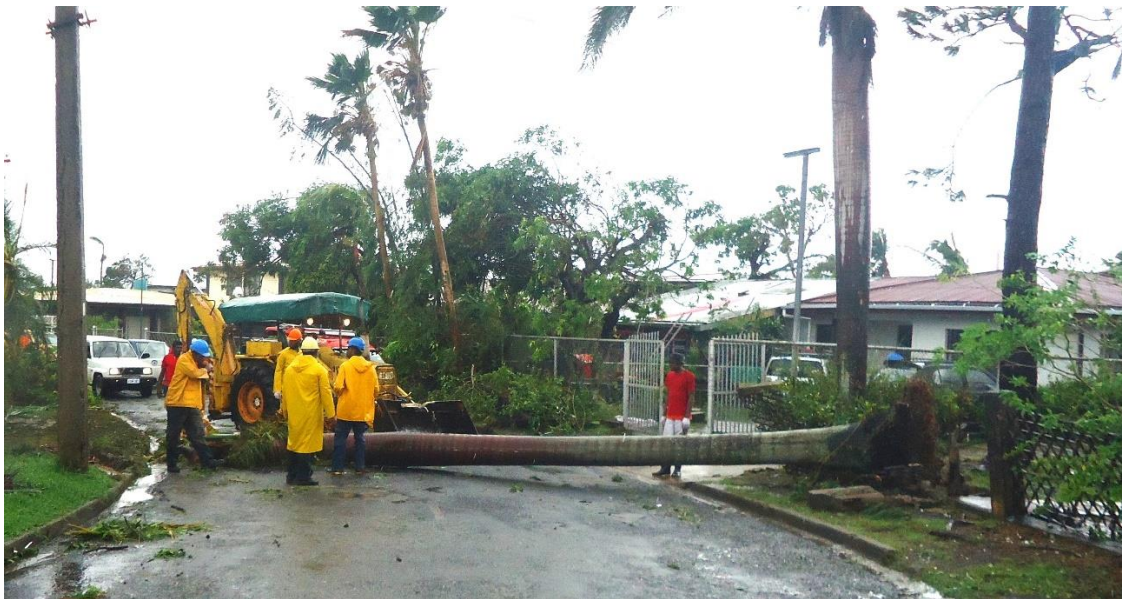
Clearing of emergency routes post disaster
